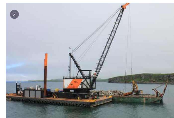
1. In-water construction had to be completed before Sept. 1 during a marine mammal window. 2. Crews completed 83,000 cubic yards of dredging on the project.
