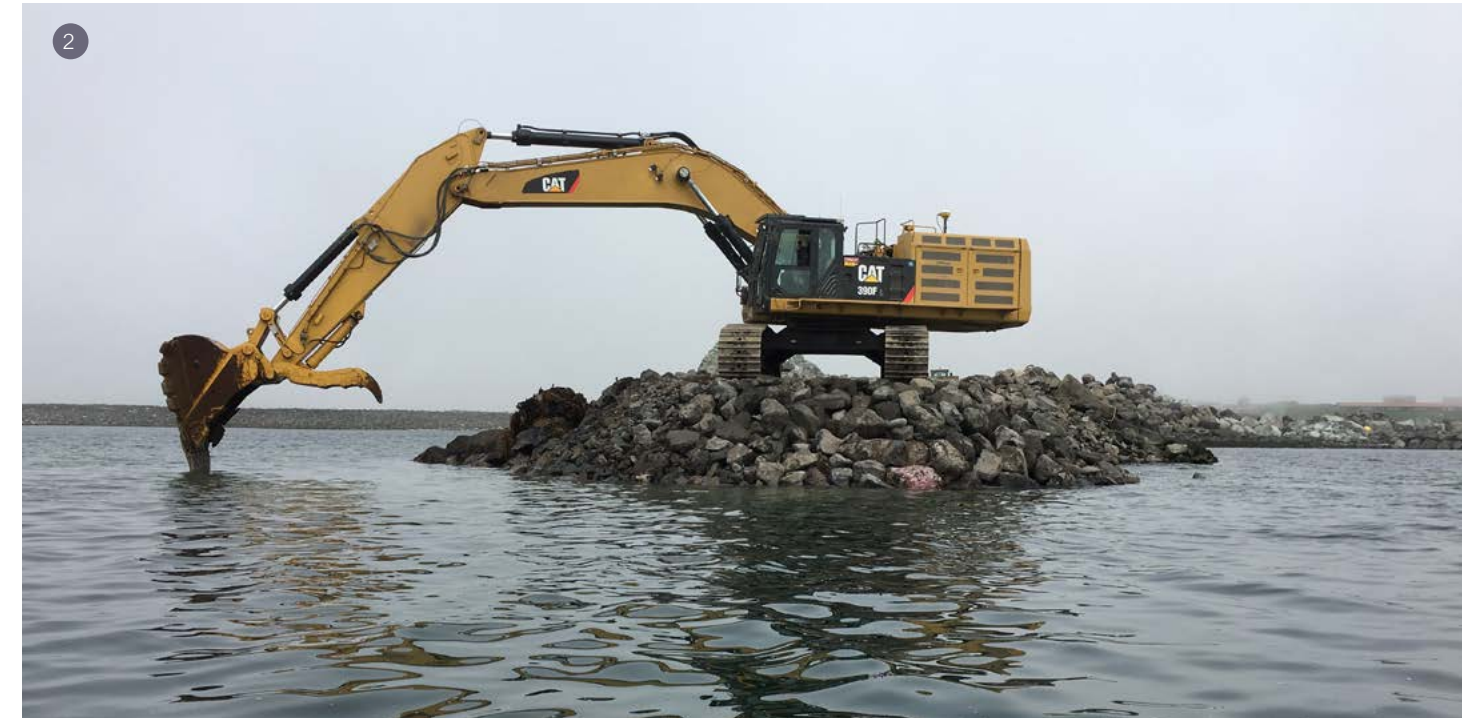
1. More than 32,000 cubic yards of armor stone and scour rock were placed on the breakwater repairs. 2. Getting the right equipment delivered to the remote island of St. Paul was an important part of planning logistics.
