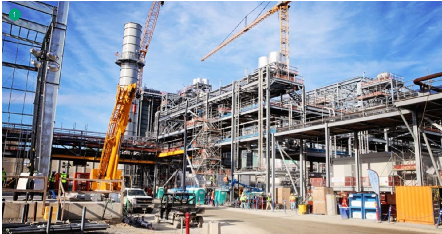
1. The power block will use two steam turbine generators to generate electricity for the facility. 2. The main cryogenic heat exchanger (MCHE) has a crucial role in the LNG process, cooling warm gas into a liquid state. 3. A centralized command center was developed to safely and efficiently manage crane activity.
