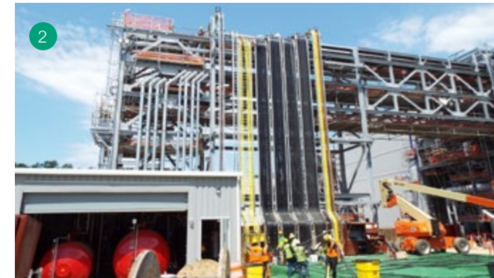
1. Crews completed expansive tabletop concrete pours safely and effectively. 2. Project controls technology was used to coordinate work and increase productivity.
