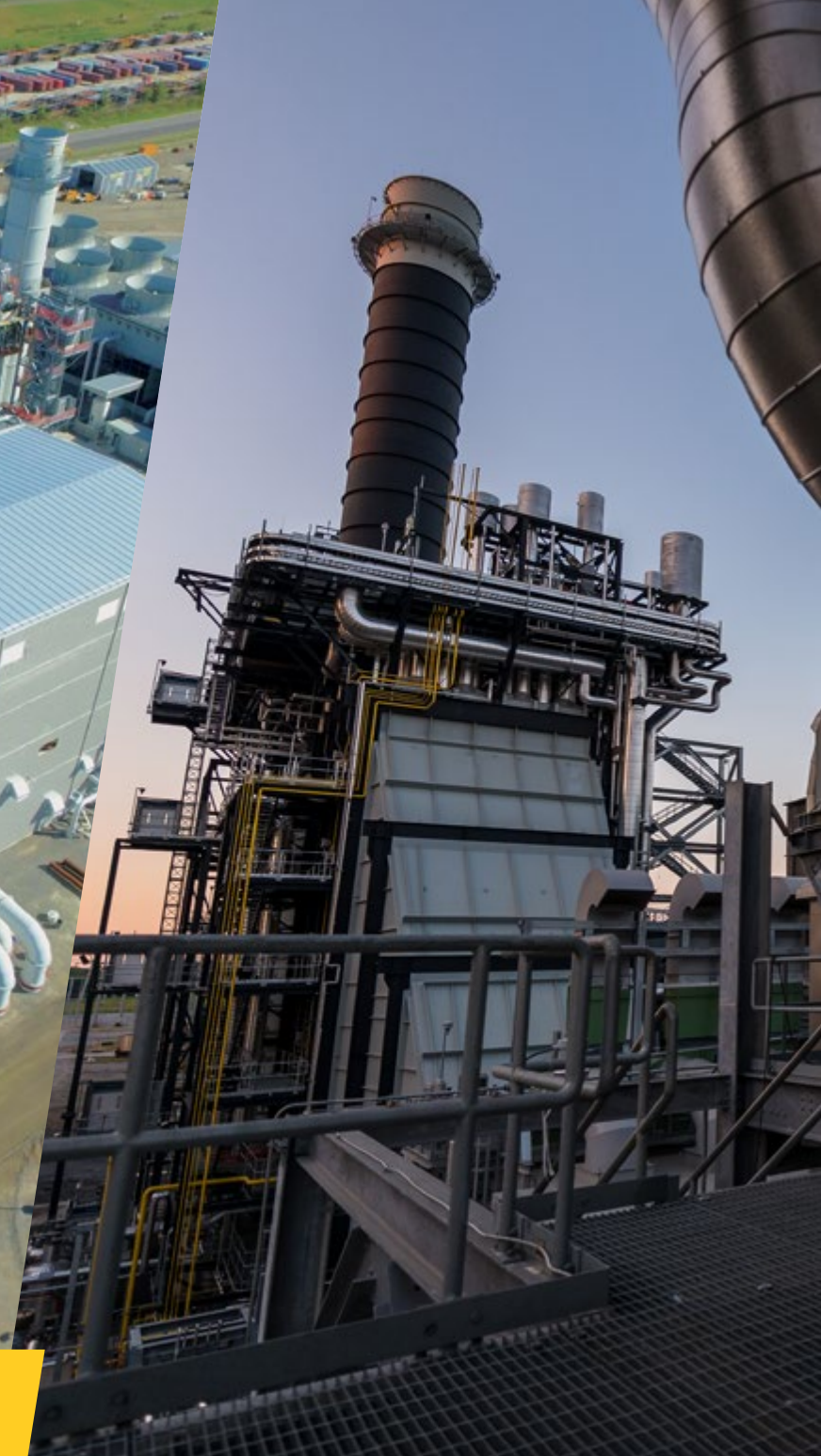
GRAND RIVER ENERGY CENTER
