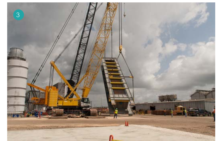
1. Increased productivity was achieved by constructing sections of the cooling tower in a nearby laydown yard and then using a platform trailer and crane to set in place. 2. Access to an in-house fleet of cranes and other equipment maximized costs and streamlined the construction schedule. 3. To transport large equipment to the construction site, TIC modified nearby roads, bridges and overhead utility lines.
