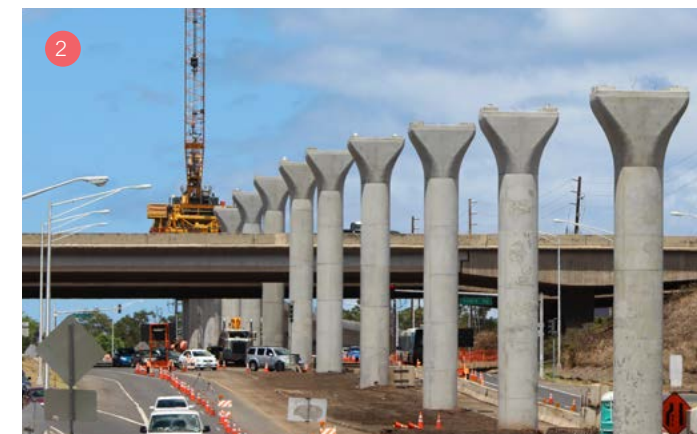
1. Crews set the final guideway segments along Farrington Highway in March 2016. 2. 450 columns were built along Farrington and Kamehameha Highways before crews could set the guideway segments on top. 3. Shaft construction along the project.
