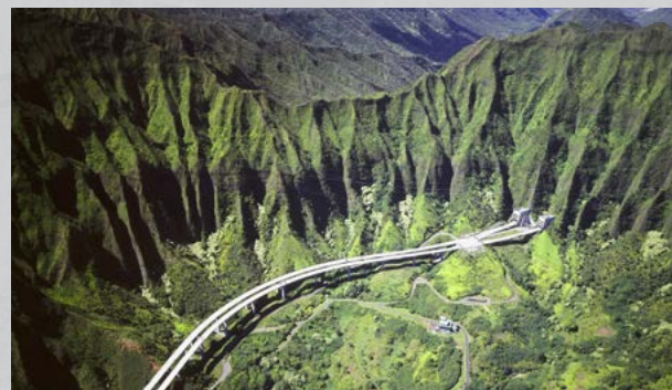
Halawa Viaducts As a portion of Hawaii's H-3 Freeway project, Kiewit constructed the side-by-side viaduct structures at the upper end of the Halawa Valley.
