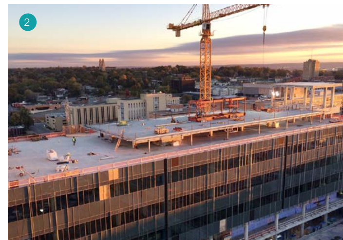
1. The Madonna Rehabilitation Hospital is a 110-bed facility that specializes in brain and spinal cord injuries. 2. A 10-story tower at the Fred and Pamela Buffett Cancer Center will feature nearly 100 state-of-the-art research laboratories.
