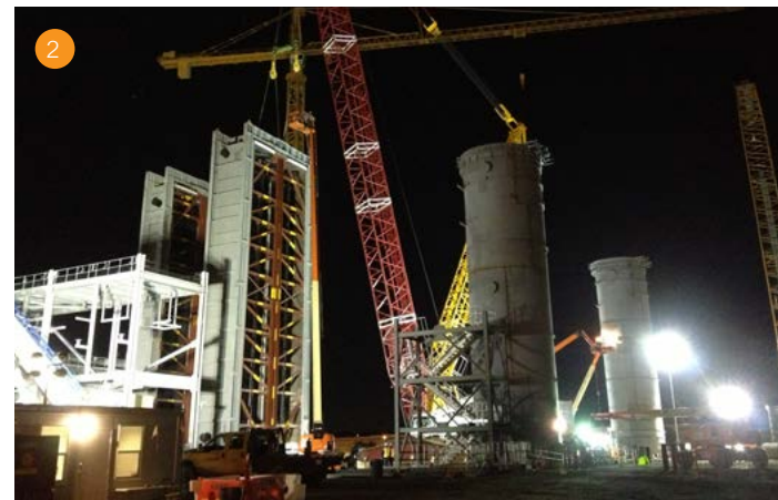
1. The heat recovery steam generators (HRSG) and pipe rack are seen as construction approached completion 2. Night crews set the HRSG modules 3. One of two GE frame 7FA.05 combustion turbine generators (CTG) installed at Woodbridge 4. The GE D11 – seen here – along with the HRSG and the GE frame 7FA.05 CTG, are all part of a Rapid Response Package from General Electric
