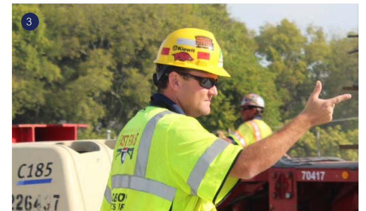
1. Precast concrete deck panels are flown into place over the CSX railroad during a weekend closure. 2. After the bridge deck is demolished, existing steel girders are picked from the original structure. 3. Project Manager Marc Rothwell was recently awarded the 2016 Peter Kiewit Award for Excellence in Management, one of Kiewit's most prestigious awards.
