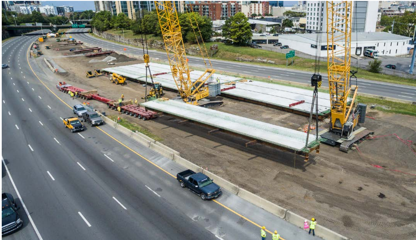
Equipment in the south yard picks panels for the Herman Street westbound bridge replacement. From there, they're set on a self-propelled modular transport that carries them to the actual bridge location, 1 1/2 miles north of the prefabrication area.
