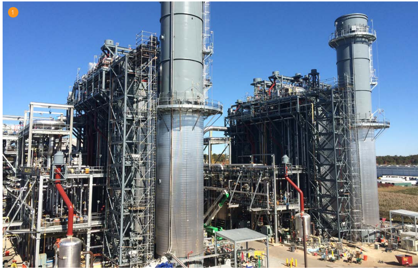
1. The heat recovery steam generators (HRSG) and pipe rack are seen as construction approached completion 2. Night crews set the HRSG modules 3. One of two GE frame 7FA.05 combustion turbine generators (CTG) installed at Woodbridge 4. The GE D11 – seen here – along with the HRSG and the GE frame 7FA.05 CTG, are all part of a Rapid Response Package from General Electric
