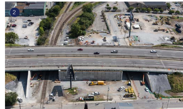
1. Kiewit's Fast Fix 8 team poses in the south yard on top of the Charlotte Avenue westbound structure. 2. Aerial view of the Clinton Street/CSX location. Innovative construction design turns an existing six-span structure into two simple span bridges.
