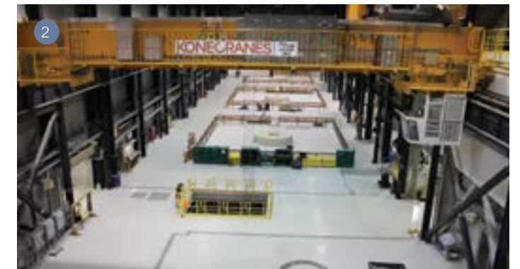
1. Aerial view of Smoky Falls Generating Station during construction (taken in 2013). 2. Inside the completed Smoky Falls Generating Station.
