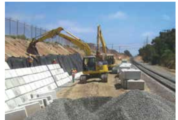
The Kiewit team built three grade crossings, installed a turnout (turning one track into two) and two crossovers (which allow trains to switch from one track to another), installed casings on about 10 utilities, excavated more than 25,000 cubic yards along the railroad right-of-way, and built two different types of retaining walls more than a mile long.
