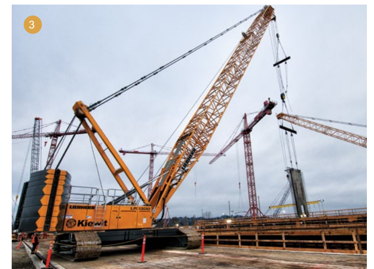
1. Crews work on a longitudinal pontoon. These pontoons are the largest, weighing 11,000 tons apiece and measuring 360 feet long, 75 feet wide and 29 feet tall. They are the largest pontoons ever built in Washington. 2. A craftsman performs a weld on a longitudinal pontoon. 3. The team at Aberdeen is constructing three types of pontoons: longitudinal, supplemental and cross.
