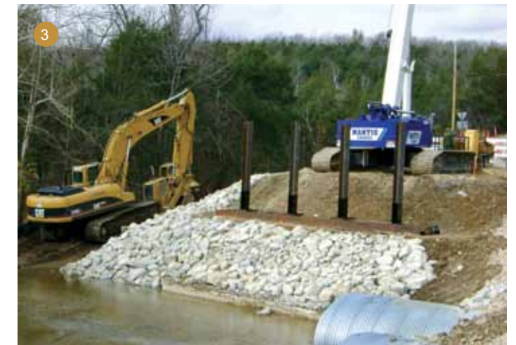
1. A 103-foot girder is positioned for a two-crane pick as part of a 311-foot-long, 30-foot-wide bridge in Christian County, Mo. 2. Ironworker crews tie wall steel in a box culvert in St. Louis. The box culvert was constructed inside an existing culvert, limiting the amount of traffic impact to 27 hours, all occurring in the evening. 3. With pile operations complete, pile cutoffs are needed to start substructure concrete. By using a 50-ton Mantis crane to drive pile, costs for mobilization, assembly and disassembly were reduced.
