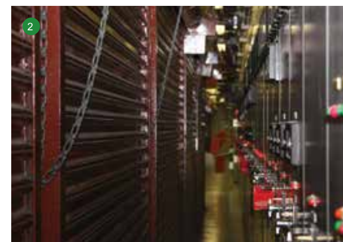
1. Pipefitters prepare to attach the base plate to the main steam line — part of the project's cooling circulating water (CCW) scope inside the plant's containment structure, nicknamed the can. 2. Inside this 4,160-volt switchgear room, large breakers feed power to equipment throughout the plant.
