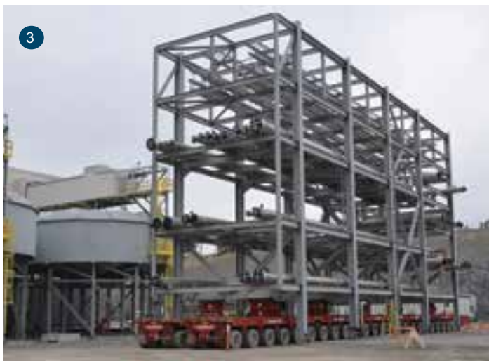
1. The massive Long Harbour nickel processing plant includes 10 separate buildings, all with a different function. 2. When all is said and done, more than 125 tanks will have been installed. Many of them require multi-crane lifts in tight quarters. Kiewit Engineering Co. has been instrumental in the design of some of these lifts. 3. Each of the plant's 10 buildings are connected by pipes, which are supported by large racks. The material moves through the pipes from station to station until there is a final product.
