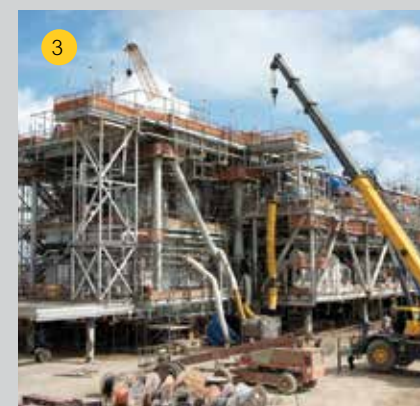
1. The Heavy Lifting Device at the Kiewit Offshore Services yard in Corpus Christi, Texas, can lift up to 11,000 tons of topsides into place at once. 2. The Shell Olympus floating tension leg platform will produce 100,000 barrels of oil per day. 3. Olympus' 25,000 tons of topsides will include living quarters, a helipad and the entire platform's control center. 4. The Noble Tamar deck is part of a 10,000-ton platform.
