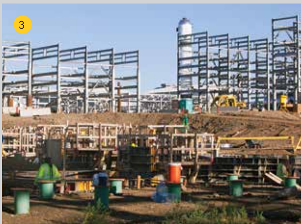
1. A crane operates at the Tioga gas processing facility in Tioga, N.D. 2. Kiewit is working to expand Tioga's processing capacity to 250 million cubic feet of gas per day. 3. With tight working quarters, the engineering team at Tioga — and its advanced use of 3-D modeling — has played a huge role.
