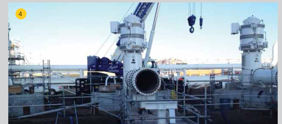
1. The Enbridge Terminal in Alberta is a major hub for oil distribution from northern Alberta oil production facilities — part of the downstream sector of the OGC market. 2 and 3. MugaFab, a company owned by Ganotec, has pipe fabrication shops in Quebec and Edmonton. 4. Fabrication of process pipe, structural steel fabrication and erection of pipe rack steel were all included in Ganotec's scope on the Enbridge Terminal.
