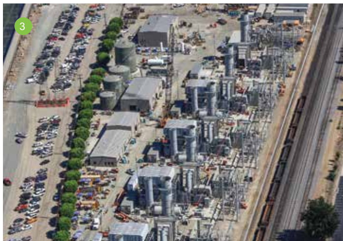
1. The Walnut Creek Energy Park is a brand new, 500-megawatt power plant for the City of Industry, Calif. It can deliver its energy to the grid within 10 minutes. 2. Craft work on the Marsh Landing Generating Station, which will provide power to 750,000 homes during peak times. 3. The Walnut Creek Energy Park was built in tight quarters. The project team had to develop a plan to minimize the impact on a congested site with a tight schedule.
