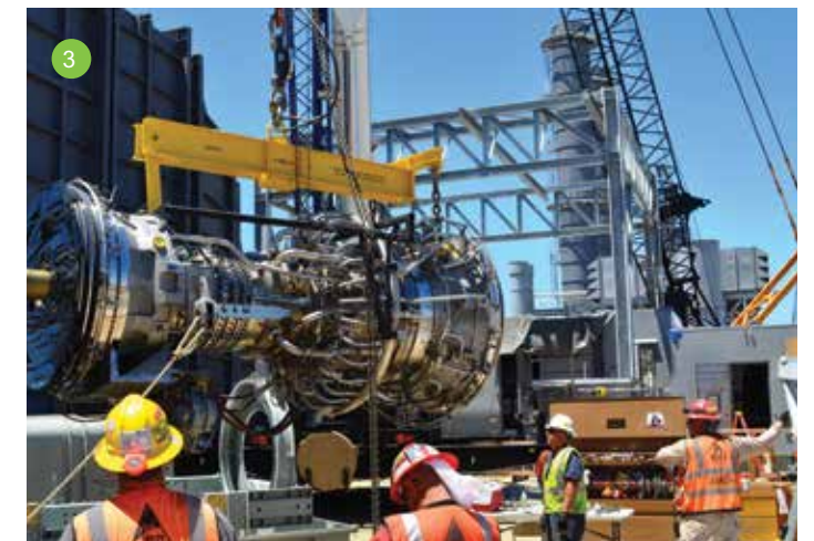
1. Kiewit built a new power plant at the Haynes Generating Station in Long Beach, Calif., to replace two older generating units. The new peakers are more energy efficient and create fewer emissions. 2. The Marsh Landing Generating Station in Antioch, Calif., can deliver 400 megawatts of energy to the grid in just 10 minutes. 3. A module is lifted into place at the Haynes Generating Station. The new units at Haynes will use a dry-cooling system as LADWP eliminates ocean cooling in its plants by 2029.
