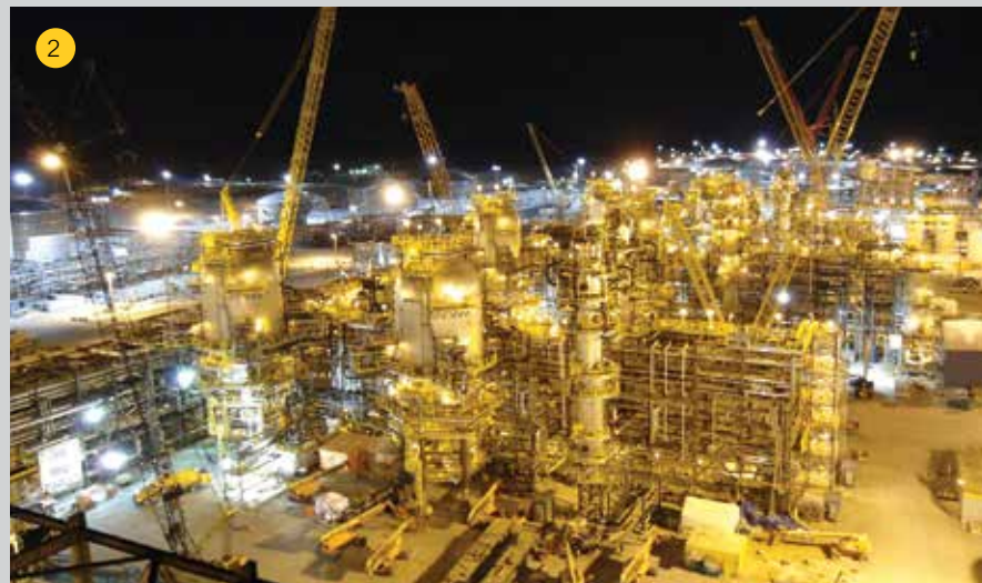
1. There are 173 billion economically recoverable barrels of oil located in Canada’s oil sands — 15 percent of the world’s oil reserves. Kiewit has executed more than $2.3 billion worth of grading and industrial work at the oil sands in Alberta. 2. Kiewit reassembled 39 modules and fabricated 900,000 feet of pipe at the Kearl Froth Treatment Silo in Alberta.
