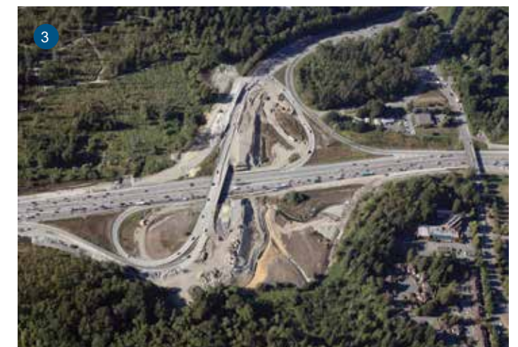
1. Bridge deck installation continues at the new Port Mann Bridge. The bridge deck, along with the cables and paving, was completed in 2012. 2. Segment 4 of the highway project included building an overpass over 152nd Street in Surrey, which is British Columbia's second-largest city by population. 3. The Port Mann/Highway 1 Improvement included the replacement of nine highway interchanges throughout all segments of the project.
