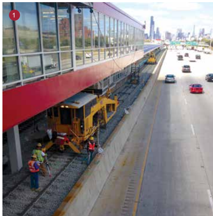
1. The Kiewit crew tamps the new track 2. Project Sponsor Mike Breyer talks with participants in the Building Tomorrow's Workforce program to discuss transit construction fundamentals and what Kiewit expects from its craft labor force.
