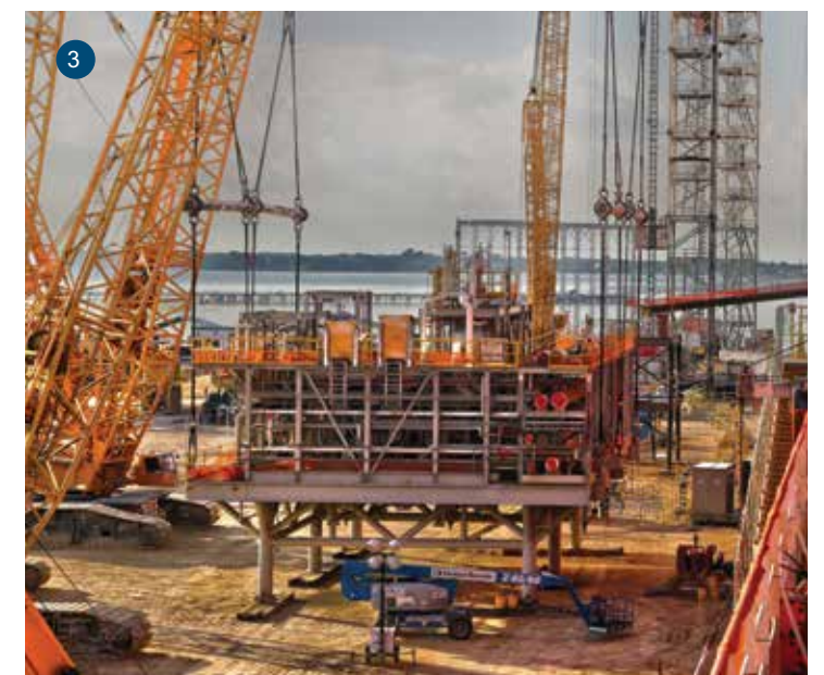
1. The riser turret module, weighing more than 700 tons, is lifted by three cranes and installed onto the modular capture vessel. 2. The project team designed and built steel module transport frames that allowed the 15 modules to be moved throughout the construction phase. 3. A processing module is prepared for the lift onto the modular capture vessel.
