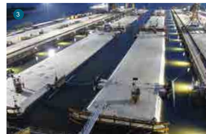
1. Workers at the Sparrows Point, Maryland, dry dock complete the first six of 11 concrete tunnel elements. The blue steel frames, called the main form traveler (left) and the egress form traveler (right), are used to form the concrete into the element shape. 2. Construction on tunnel elements 3, 4, 5 and 6 is completed in dry dock. 3. Flooding of the Sparrows Point dry dock began at the beginning of June 2014, with the elements towed one-by-one to Virginia.
