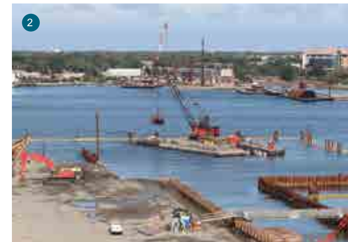
1. As Element 1 arrived in Virginia, workers secured the tunnel element with lines to a Portsmouth wharf along the Elizabeth River. Immersion of the first element is scheduled to occur in late September. 2. Work continues on the Portsmouth side of the Elizabeth River — the crane situated on top of a barge is dredging to prepare for the immersion of the first tunnel element. 3. An aerial view of the Elizabeth River Portsmouth approach for the new Midtown Tunnel.
