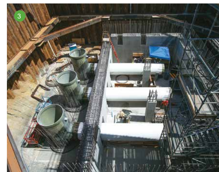
1. Employees work on setting forms for chemical tank pads in what will be the plant's chemical storage area. 2. In addition to solar panels, 12 kilovolts of power will energize the desalination plant. 3. Three vertical turbine pumps at the intake pump station will feed 100 million gallons of water a day into the plant. 4. Two KSD employees discuss the progress of the pipe rack, left. The rack will support pipes ranging from one to 72 inches.
