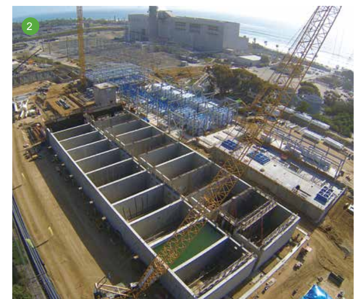
1. Up to six cranes were in use at one time during construction. 2. Designer IDE typically designs plants like Carlsbad on 25-acre lots. Carlsbad has been designed for and is being built on only seven acres.
