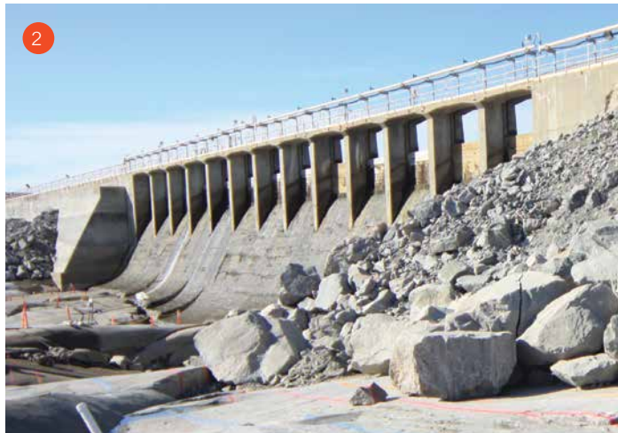
1. 100-year-old dam structure awaiting decommissioning. 2. Section of the old dam sealed with oakum to allow clay core dam construction to begin.
