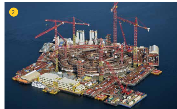
1. In June 2014, more than 1,500 people celebrated 10 million manhours without a lost time incident at the Hebron GBS. 2. The GBS and surrounding flotilla seen from above at the deep water site. The flotilla includes a floating concrete batch plant.
