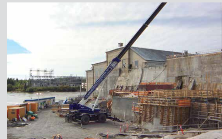
Construction of the powerhouse tie-in wall with the 1912-built powerhouse in the background.
