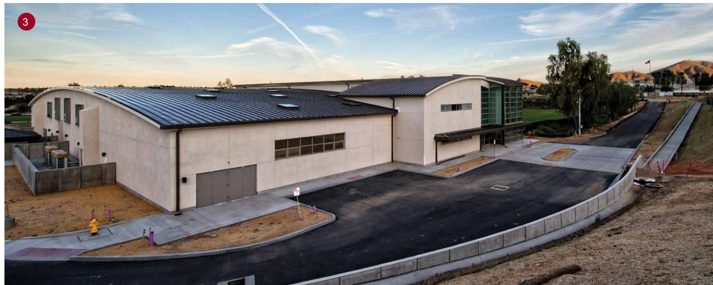
1. The Easton Archery Center of Excellence features windows that, when opened, can double as a progressive training tool. Archers can stand inside the building and shoot at outdoor targets. 2. Lexan windows will provide spectators crystal clear, protected views of archers in the shooting room as they walk through the center's hallways. 3. An overview of the Easton Archery Center of Excellence.
