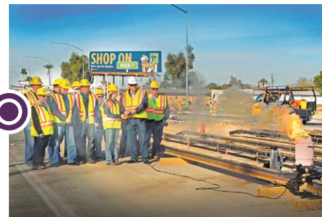
FEBRUARY 2014 First rail weld milestone event
