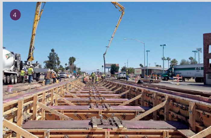
1. Crews prepare to set the electrical vault base for the light rail line's electrical system. 2. A trench is formed to prepare for the installation of the communication ductbank. 3. An operator unloads 80-foot strands of rail. 4. VTC places concrete for one of four station platforms that are included in the extension. 5. Crews pull communication lines from a manhole along the Central Mesa Extension.
