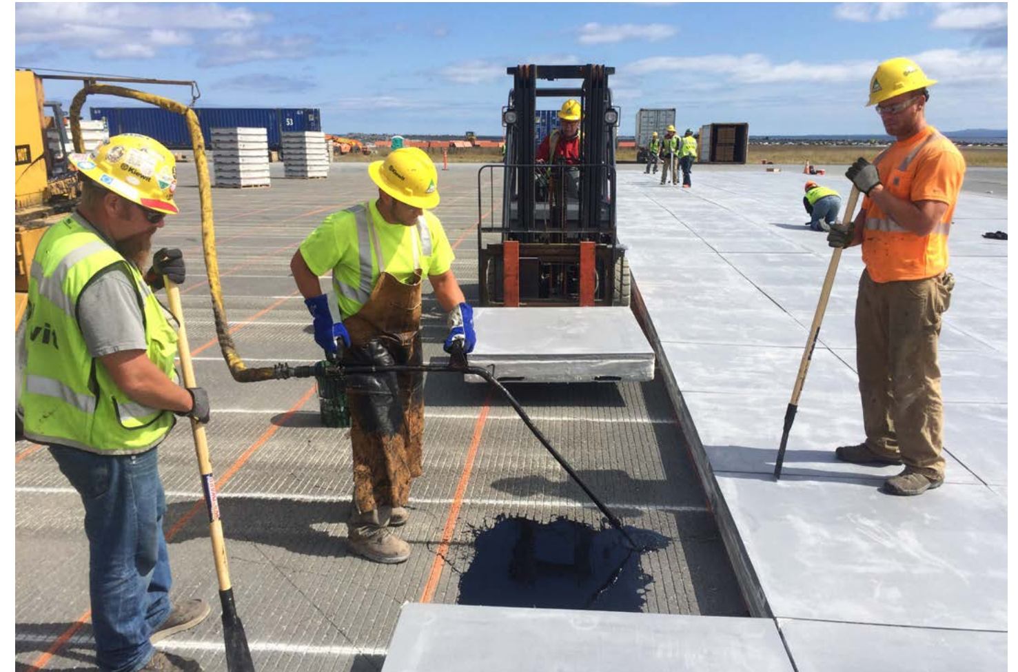
Crews install EMAS blocks at Kodiak Airport. These were the first EMAS bed installations by a Kiewit company.
