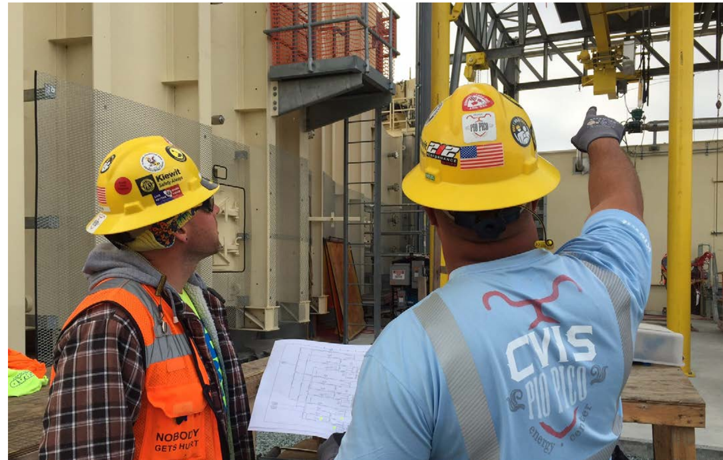
Instrumentation fitters at the Pio Pico Energy Center discuss access plans and how they’re going to prevent dropped objects from occurring during their operation.
