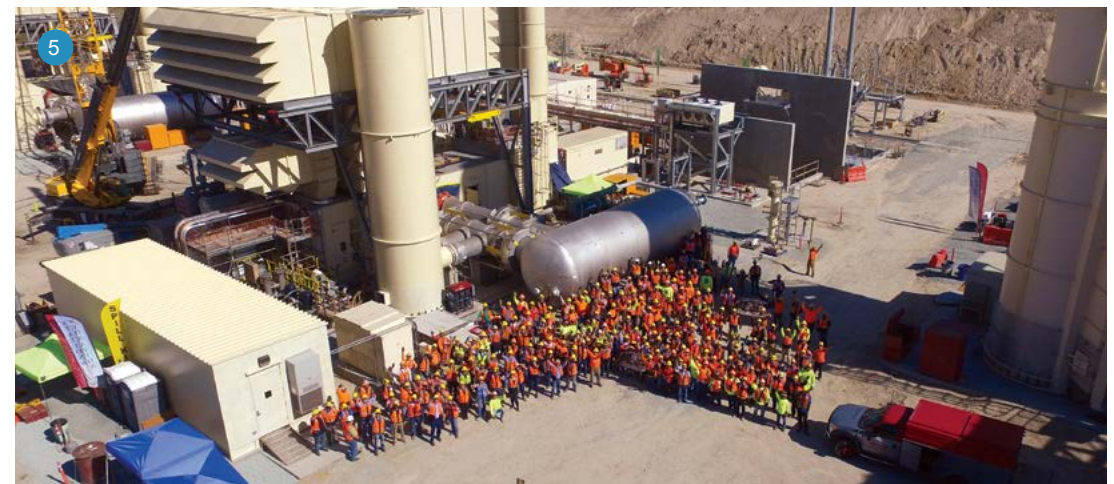
1. Combustion turbine units 1, 2 and 3 are seen from overhead at the Pio Pico Energy Center project. 2. Construction is a coordinated effort between many moving parts, as seen in setting the unit 3 inlet air filter at Pio Pico. 3. Crews place exhaust stack anchor bolts. 4. A network of electrical ductbank is seen in the main trench on the site. 5. Team Pio Pico poses proudly for a team picture in January 2016.
