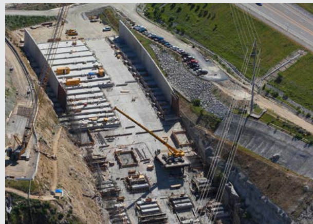
Step chute: Dropping water over 160 feet in elevation, the structure is stepped to help dissipate the energy of the water coming downhill. A special concrete mix is used to prevent scouring and erosion.
