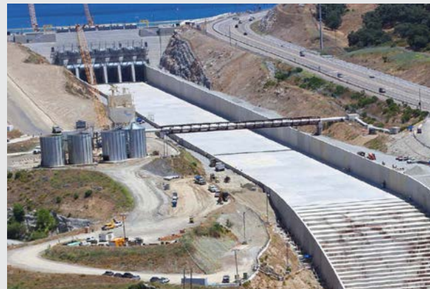
Upper chute: A little over 2,000 feet long, the upper chute tapers downhill at a two percent grade.
