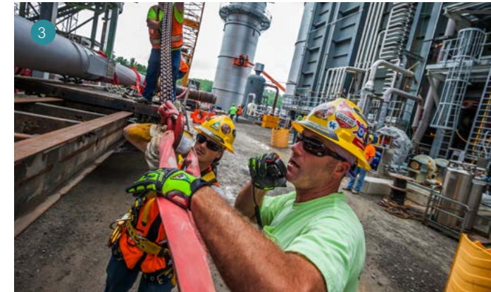
1. Dawn at the Paradise Combined Cycle Plant 2.-3. Boilermakers hanging rigging on the crane hook in preparation to install pipe in the unit.
