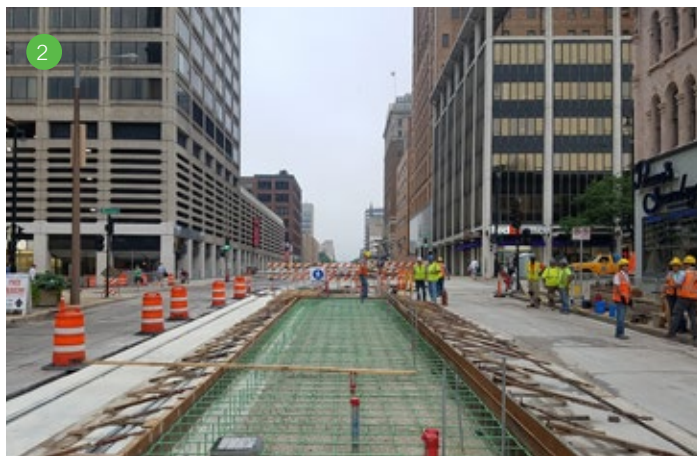
1. Pedestrian control was a foremost concern during construction, particularly in areas such as the Historic Third Ward, a revitalized warehouse district filled with shops and restaurants. 2. Construction of a station platform is completed in the center of downtown Milwaukee. 3. Prepour checks are performed by Kiewit staff prior to every concrete pour.
