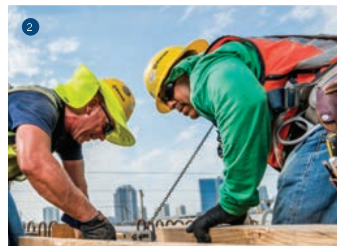
1. Pier caps for the HOV flyover structure. 2. Carpenters build formwork for a cast-in-place soffit. 3. Planning Manager Chris Miske walks through the next day’s planned work at the Play of the Day meeting.
