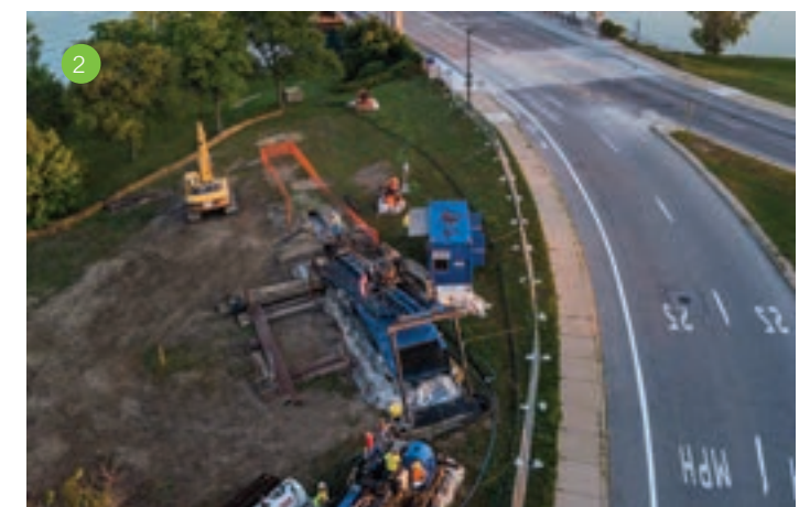
1. The majority of power lines in the U.S. were installed 60 or 70 years ago, operating beyond their intended life cycle and in need of replacement. 2. Using horizontal directional drilling, Kiewit is installing new underground distribution lines as part of a major renovation project along the Detroit River.
