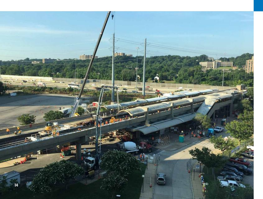
Kiewit's task: remove the old edges and replace them with new, structurally sound edges.
