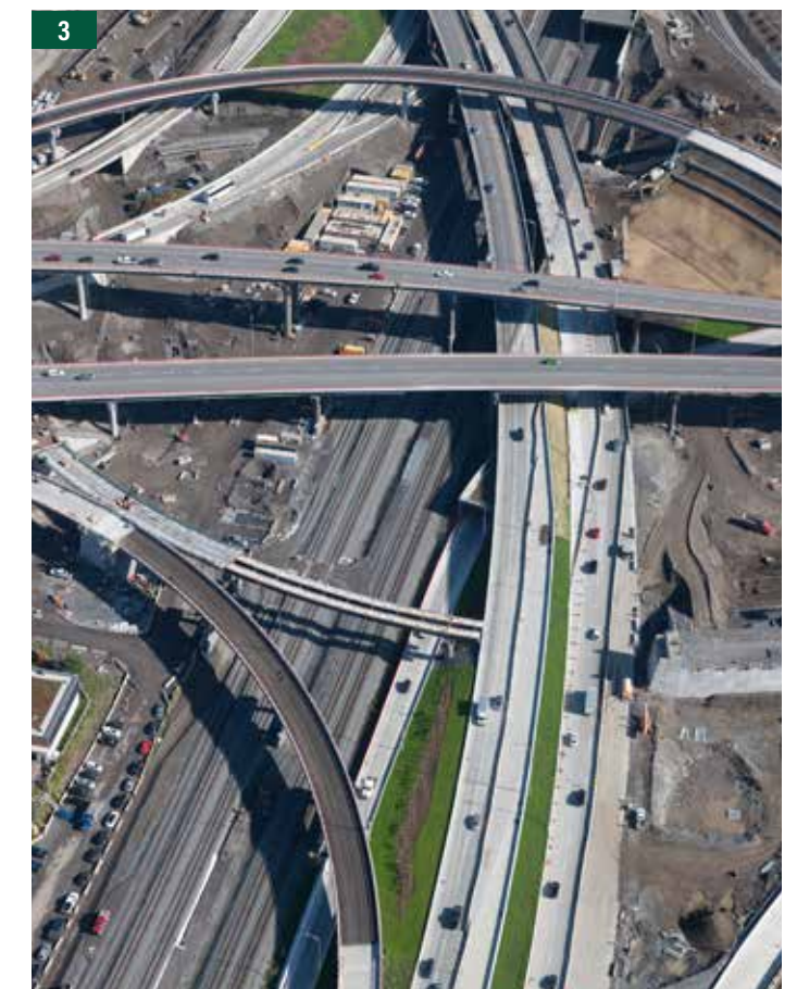
1. The old ramp from Highway 20 East toward Highway 15 North was dismantled to make way for the new interchange. 2. A look back, this photo shows an earlier view looking east toward the former Highway 720 West. 3. An aerial view of the new ramps at the heart of the Turcot Interchange.
