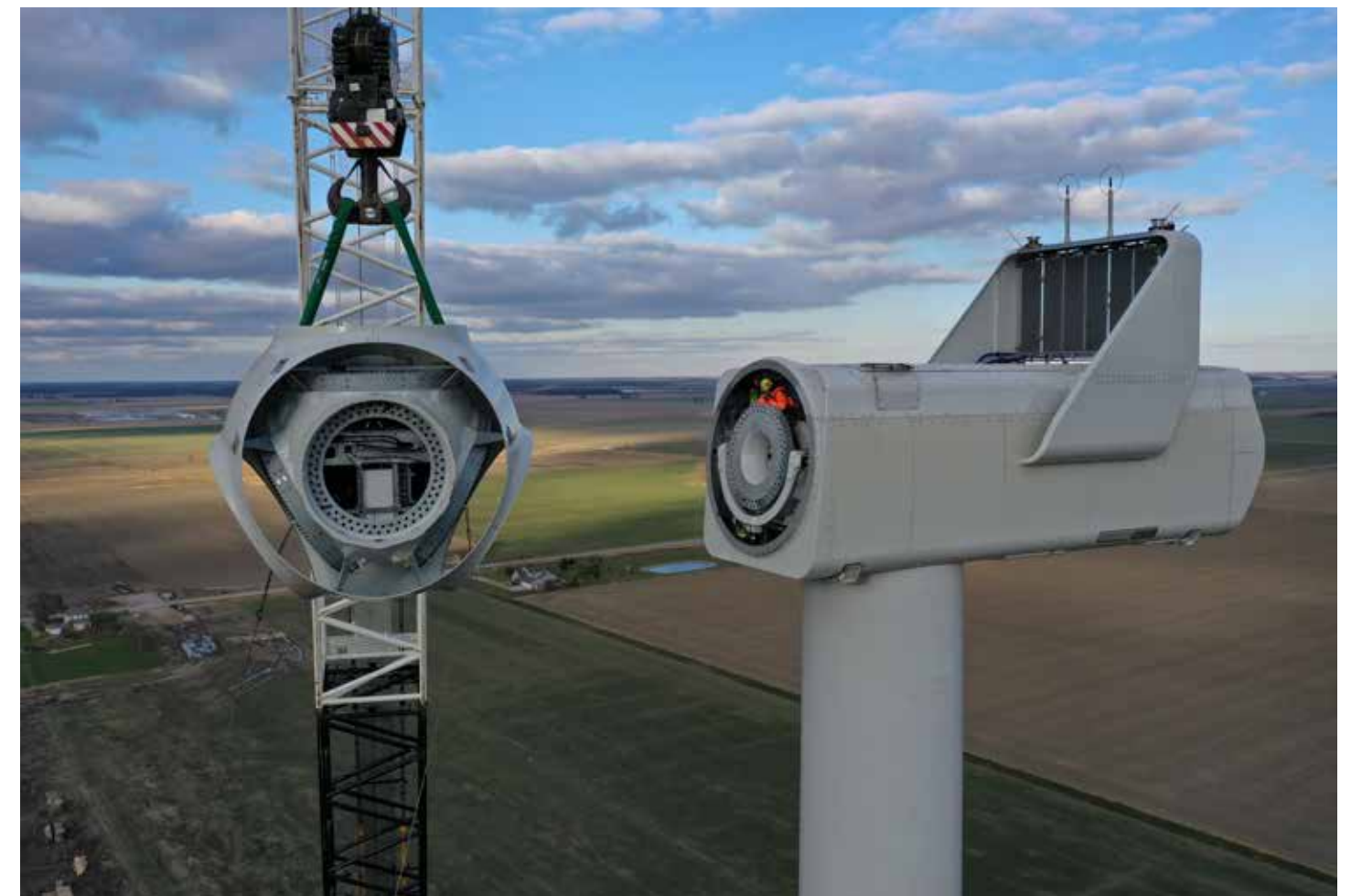
The hub of this Vestas V150-4.2 megawatt turbine is shown being set on the nacelle. The blades will be attached to the hub, which is 105 meters high.
