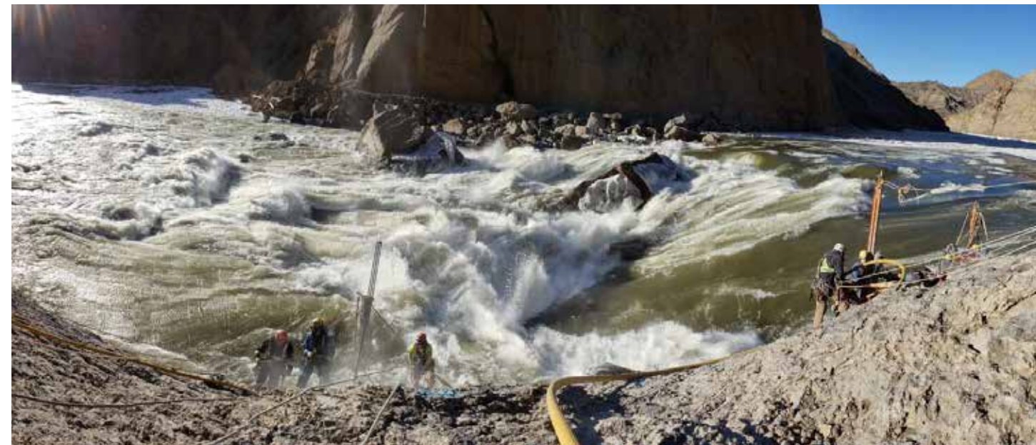
Crews drill blast holes on the East Toe for channel constriction widening.
