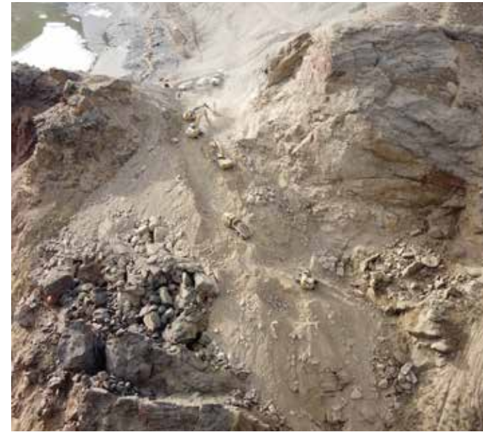
Crews drill, excavate and work on embanking the access road in the through cut.
