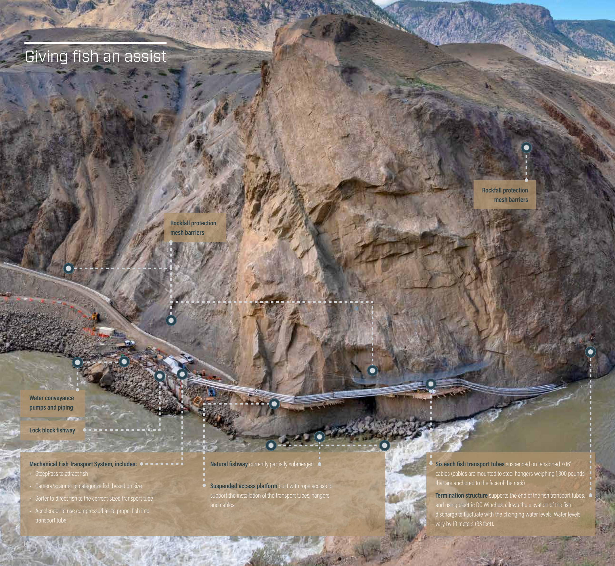
Rockfall protection mesh was pinned on the brow of the slide area to protect the team (paint marks in the photo show completed pins).
