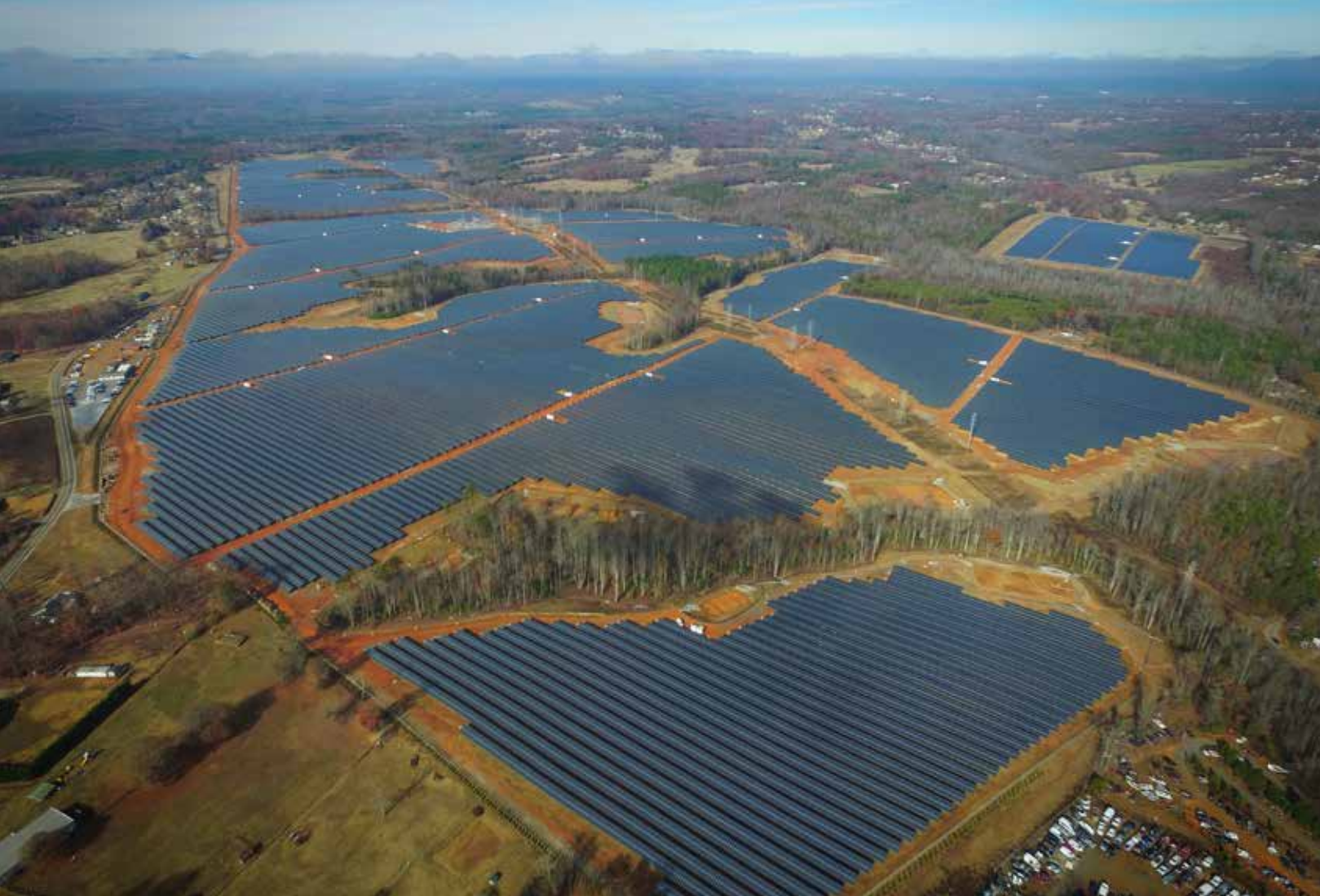
MEC installed conduit, cable and electrical equipment for nearly 300,000 solar modules on the 480-acre Rutherford Solar Farm in North Carolina.
