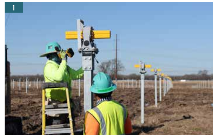
1. Slew drive tracker systems are installed to turn panels throughout the day to receive the maximum amount of sunlight. 2. Boxes of panels are lined up for installation once the posts and racking systems are in place.
