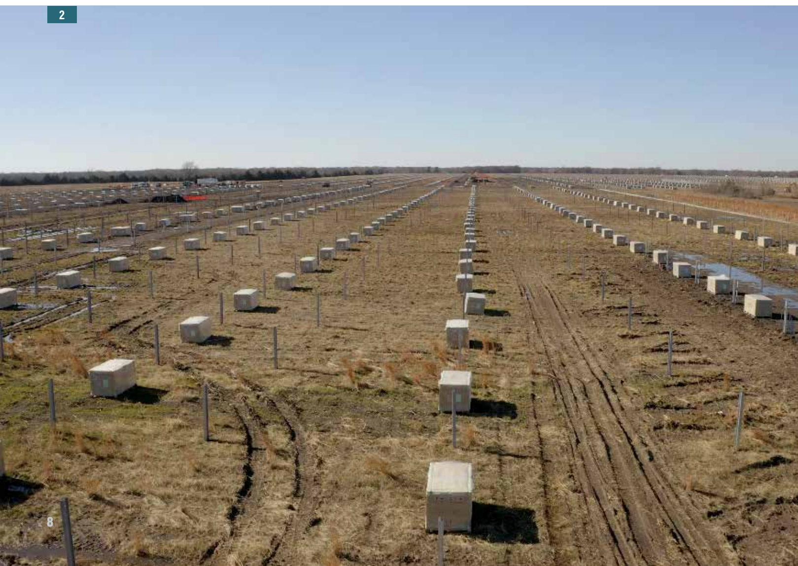
1. Slew drive tracker systems are installed to turn panels throughout the day to receive the maximum amount of sunlight. 2. Boxes of panels are lined up for installation once the posts and racking systems are in place.
