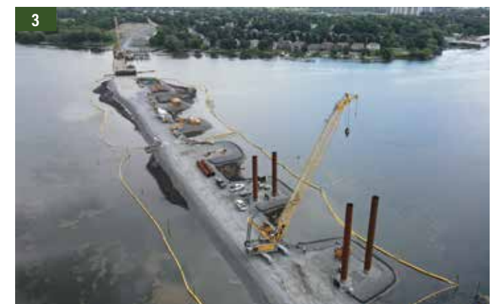
1. New Kiewit shareholders and managers in Canada visit the Kingston Third Crossing project. 2. This photo shows the first crossing of a Kiewit LR 1200 SX on the temporary trestle lift span over the Cataraqui River. 3. Driving deep foundation casing with one of Kiewit's HS 895 cranes on the temporary rock causeway.
