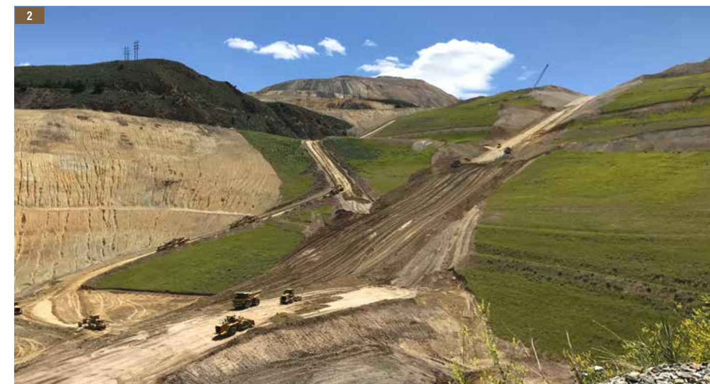
1. The Kiewit maintenance team was quick to arrive at the site of the breakdown and perform a major repair to the crawler. 2. Kiewit's scope of work included 2 million cubic yards of excavation and embankment to create new crushed ore conveyor corridors.
