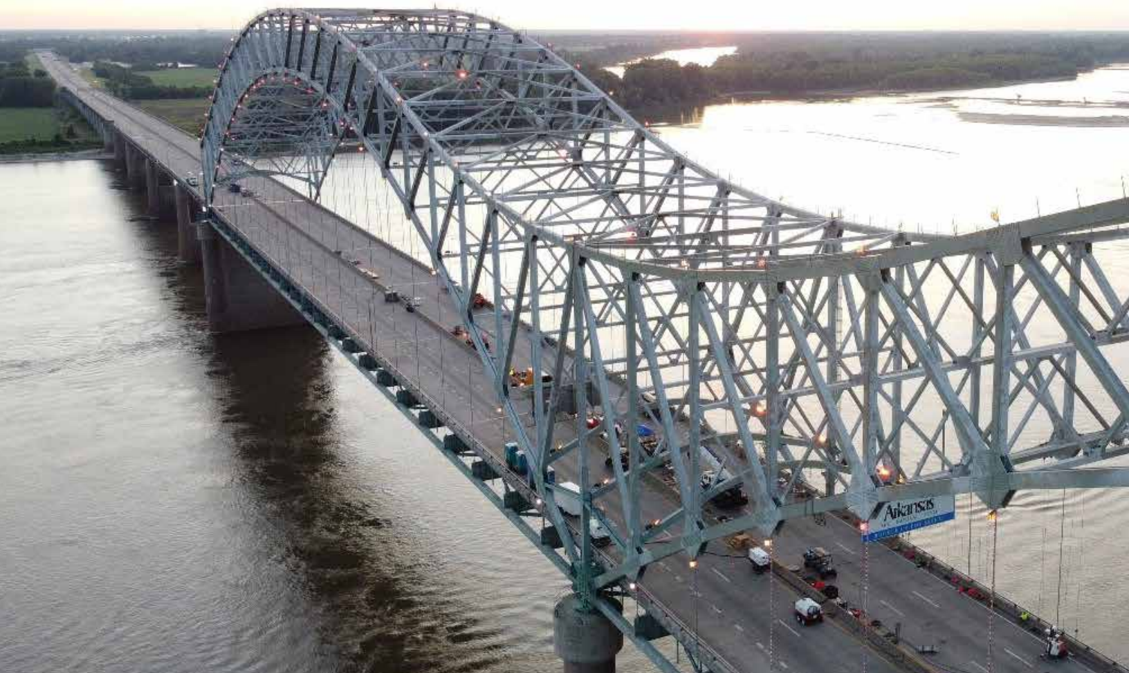
I-40 HERNANDO DE SOTO BRIDGE | MEMPHIS, TENNESSEE TO WEST MEMPHIS, ARKANSAS
