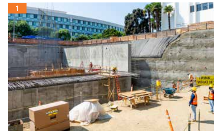
1. The Sustainable Water Infrastructure Project (SWIP) included construction of a below-grade, advanced treatment facility to treat a blend of sewer and stormwater at the Santa Monica Civic Center lot shown here. 2. The SWIP team stands in the 1.5 million gallon stormwater capture tank for a photo.
