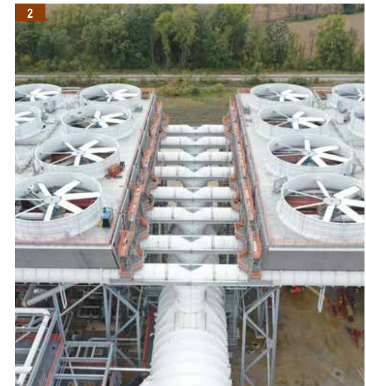
1. Crews install drilled piers to support the 345-kilovolt collector yard structures. 2. The steam distribution duct for the 47-cell Induced Draft Air Cooled Condenser (ACC) is 31 feet in diameter at its largest point. At full load, the duct distributes 2 million pounds per hour of steam to be condensed back into water.
