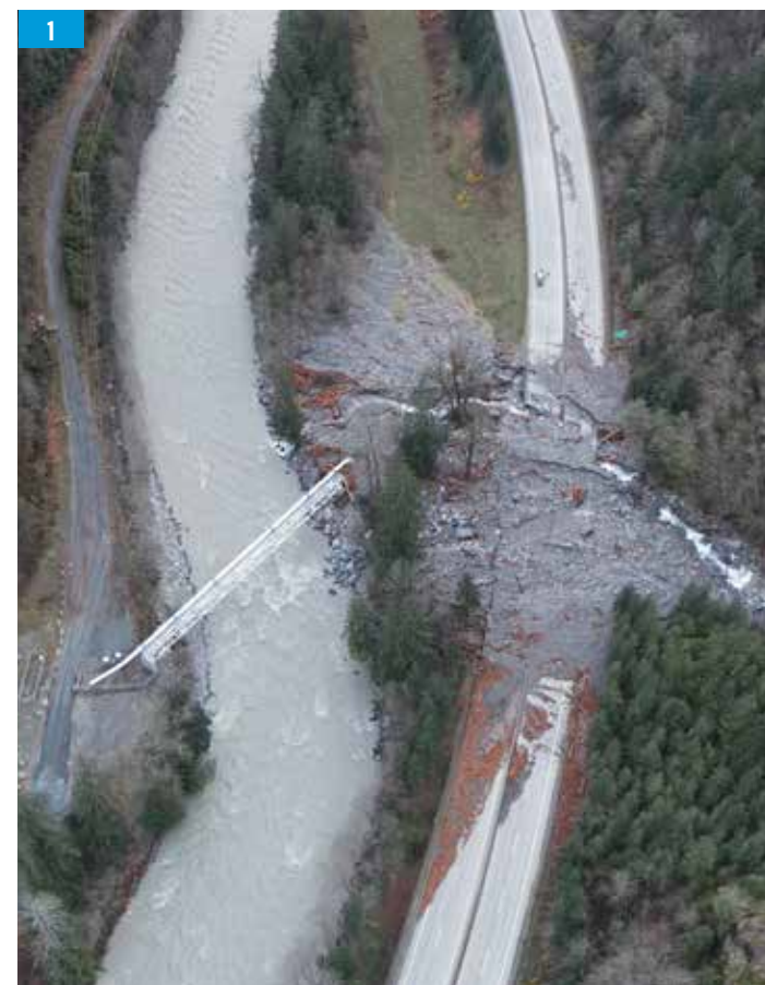
1. One of many significant mudslides on the Coquihalla Highway that made the road impassible is shown in photo 1 below. 2. This photo shows the highway after crews cleared debris and made road repairs to restore traffic. 3. Personnel relied on helicopters to reach numerous project sites that were otherwise inaccessible. 4. Kiewit employees Etienne Bossé and Stéphanie Massey supported the volunteer effort at the Hope refugee center, providing food and supplies to community members in need. 5. Kiewit Engineering Operations Director Jorge Antunes shares project plans with B.C. Ministry of Transportation and Infrastructure Engineering Director Kevin Weicker.
