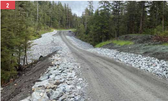
1. Crews assembled the multi plate on site in 4-foot sections due to access and transport limitations. 2. The road was constructed with materials obtained through the excavation and drill and blast process.
