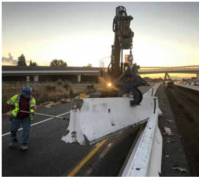
K-rail was set in place as protective barriers against the traffic that surrounded crews on site.
