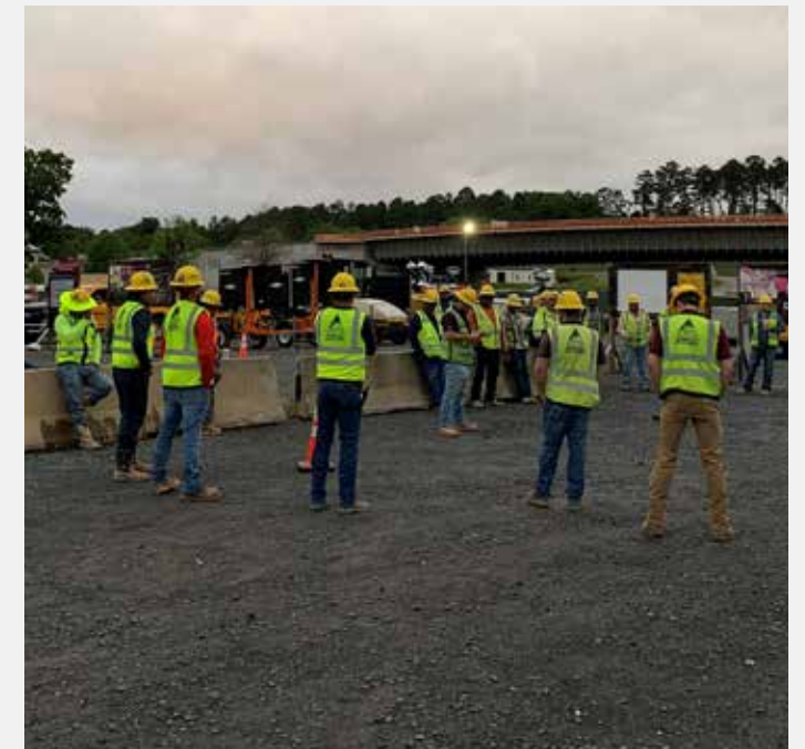
The Jack-Stone 10 project team held a demonstration of crush and pinch points mitigation techniques while handling a precast concrete traffic barrier.
