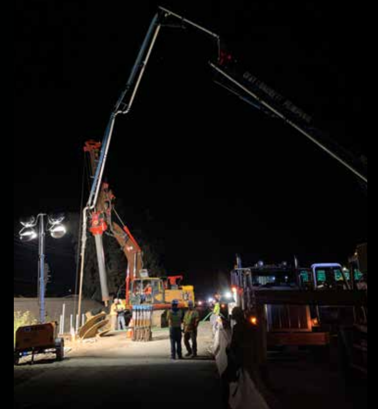
All night work was completed behind barriers with lane closures communicated well in advance.
