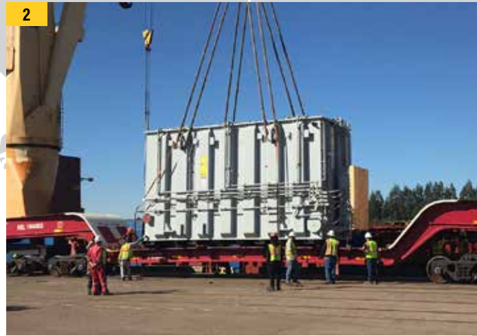
1. Kiewit employs a category management program to inform purchasing decisions across projects. 2. The generator step-up transformer pictured above was the largest unit the supplier had exported from Brazil to date.
