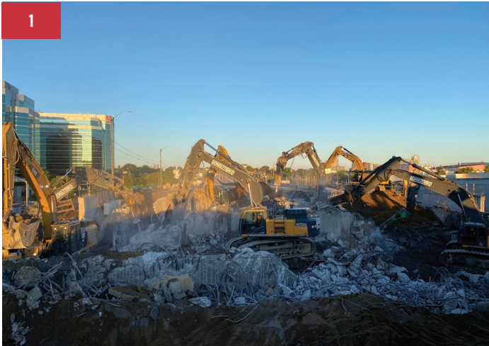
1. Demolition of the Percy St. Overpass during the rapid bridge replacement in October 2023 2. An overhead view of HWY 417 & Booth St. Overpass during construction 3. Crews at work during the ongoing paving operations 4. Booth St. Overpass Structure moving into place via self-propelled modular transporter (SPMT) during the rapid bridge replacement in August 2022
