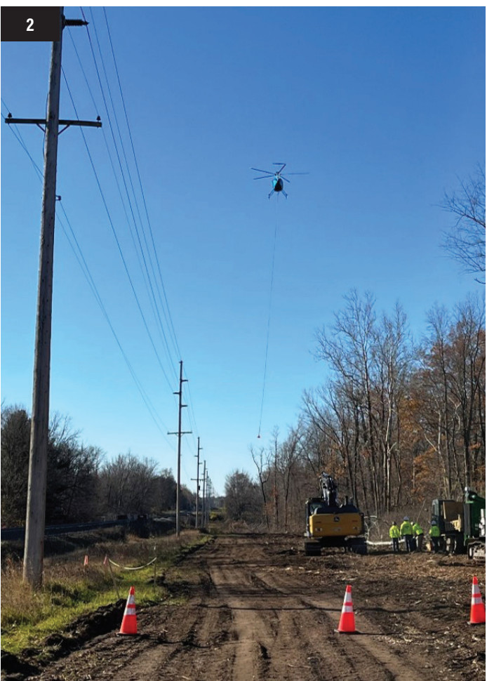
1. Power delivery requires meticulous planning and design, but still has to be carried out in the field by experienced craft workers. 2. Remote locations for transmission lines necessitate specialized equipment, including the occasional use of helicopters.
