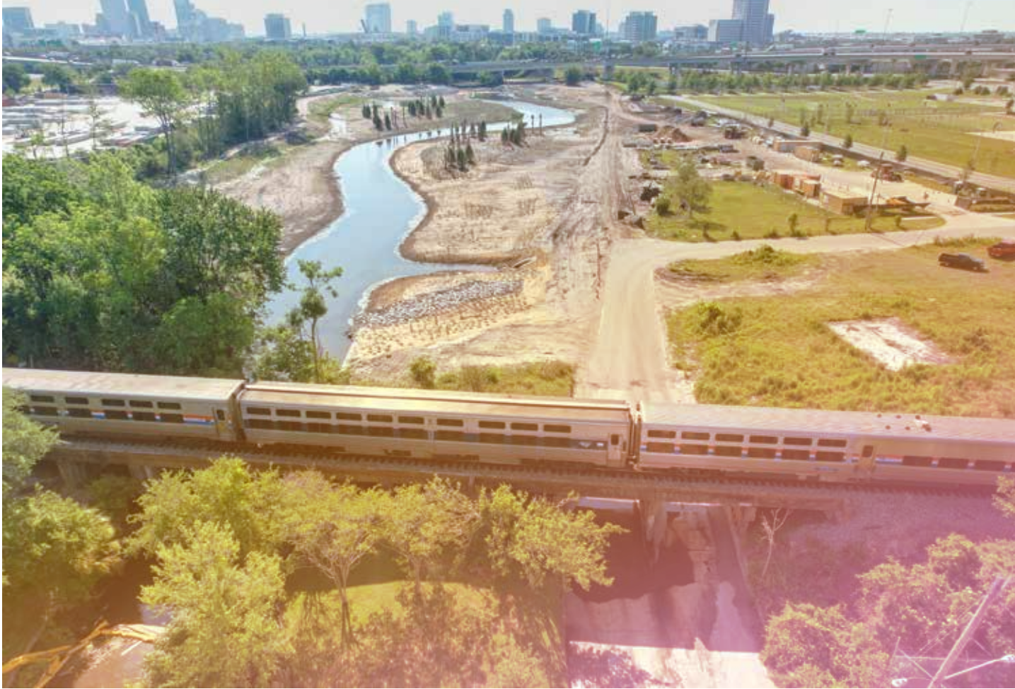
Kiewit crews replace an existing, artificial straight channel with a new, meandering channel with additional water containment areas, such as lagoons and tidal pools, to function more like a natural flood plain.
