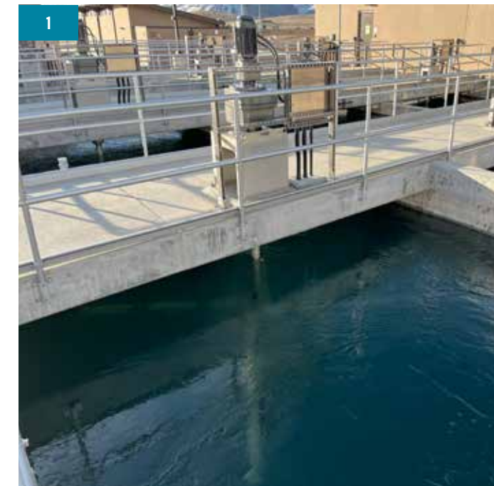
Flocculation basins (1) are connected by concrete baffle walls with sedimentation basins (2). Together, they capture and remove sediment and debris prior to filtration. Northwater features three floc-sed trains each capable of treating 25 MGD, with provisions for future expansion.
