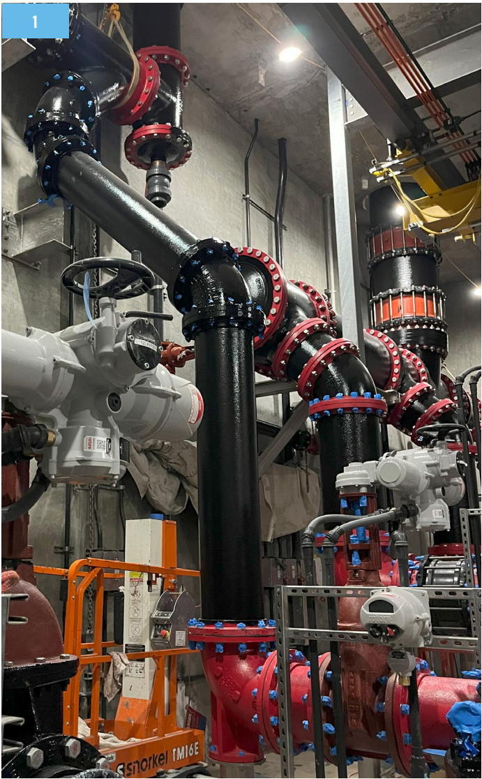
1. At the Ballona Creek facility, pumps draw water from the wet well and distribute it through two separate flow paths. One header routes water vertically through the roof to the ozone disinfection system, while the other directs flow to the Hyperion Water Reclamation Plant via a bypass line. 2. The first step in constructing the pump station buildings involved preparing the foundation. Here, the pour crew places concrete for one section of the Ballona Creek building. The foundation was covered with a vapor barrier and reinforced with rebar and concrete forms, ensuring long-term stability, preventing groundwater seepage and maintaining building integrity.
