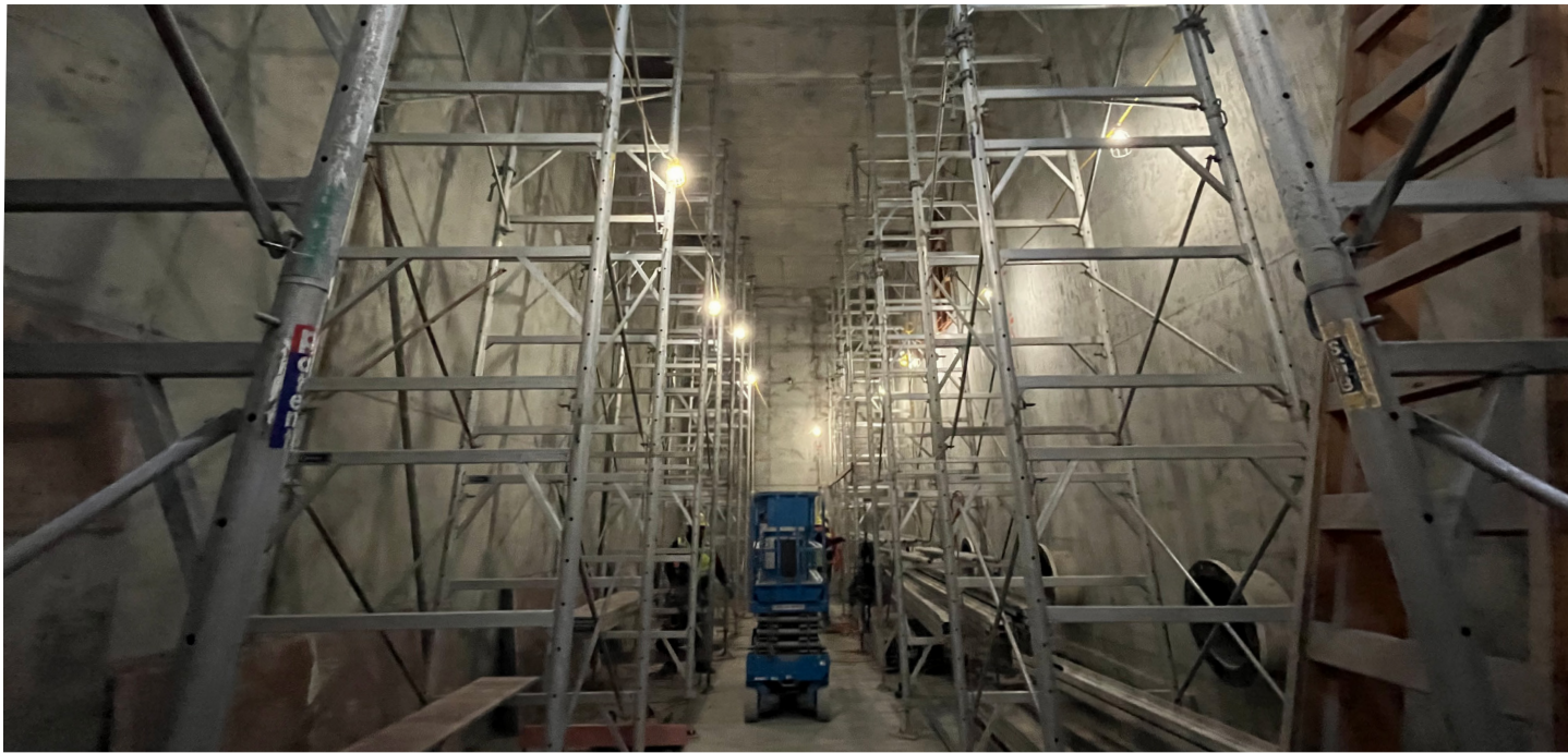
Falsework towers were used to support a deck inside the wet well at the Ballona Creek Pump Station. The wet well is where all stormwater runoff from Ballona Creek is collected before being pumped through the ozone disinfection system.
