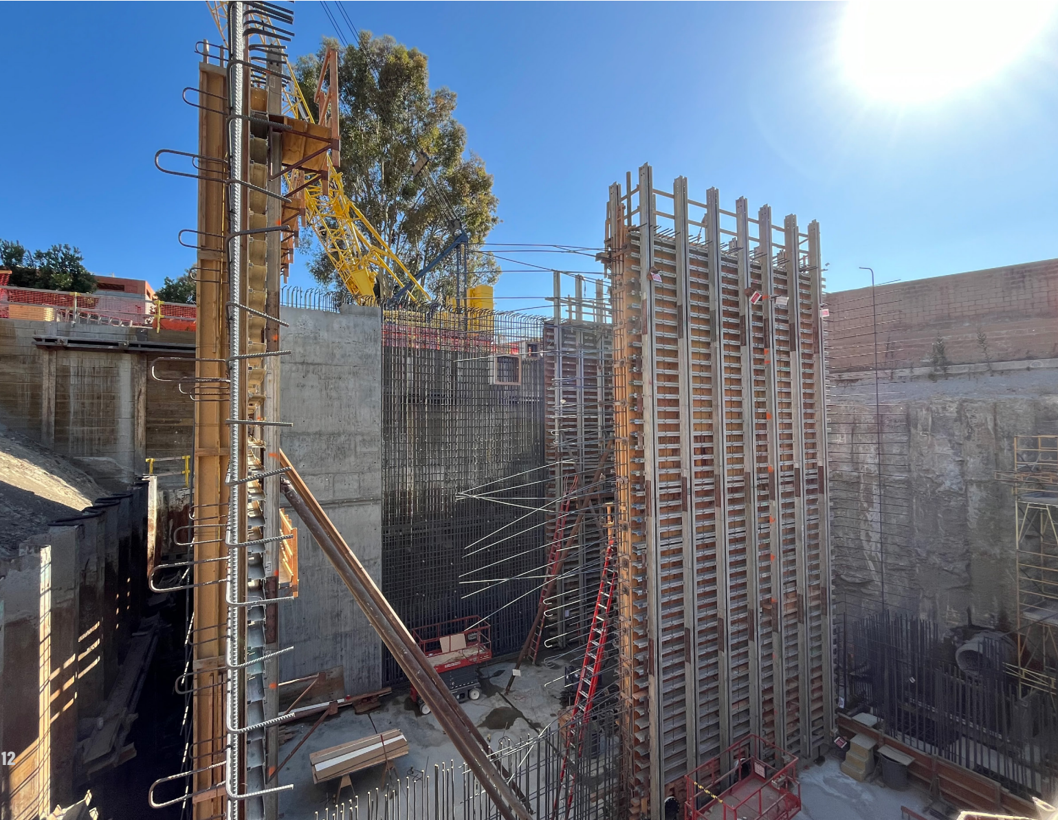
It’s no small feat constructing 50-foot concrete walls. This progress photo at Ballona Creek, taken at about 15 percent completion, shows two corners of the building being poured as crews erected the next two wall sections. Maintaining the design pour rate was vital to prevent formwork failure.
