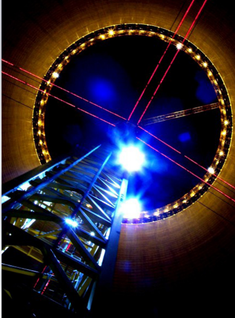
The LR 1300 SX operated inside the Brayton Point Closed Loop Cooling tower in Somerset, Massachusetts, where Kiewit engineered, procured and constructed a 1,575-megawatt conversion from open-to closed-cycle cooling. Completed in 2013, the project also added a new substation to improve efficiency and environmental performance.
